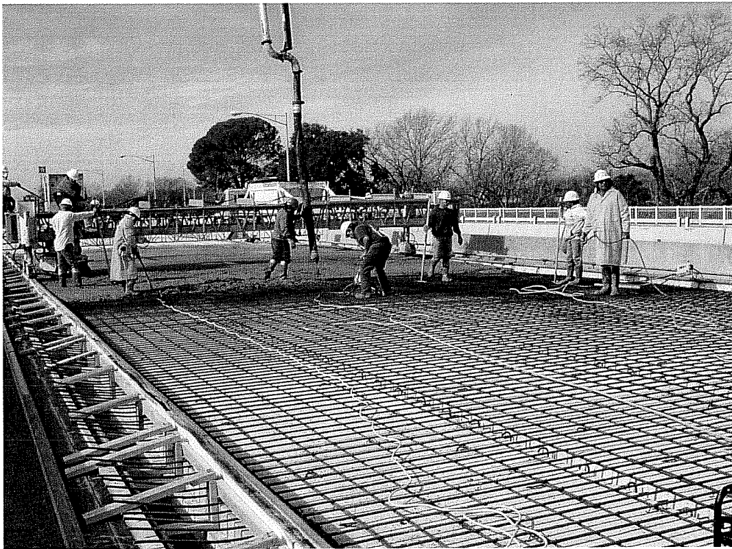
Figure 1.7 Placing concrete in the field (Ryan 2003)
