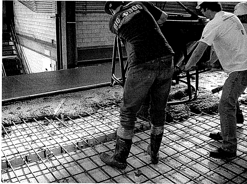
Figure 4.7 Placing the topping slab
