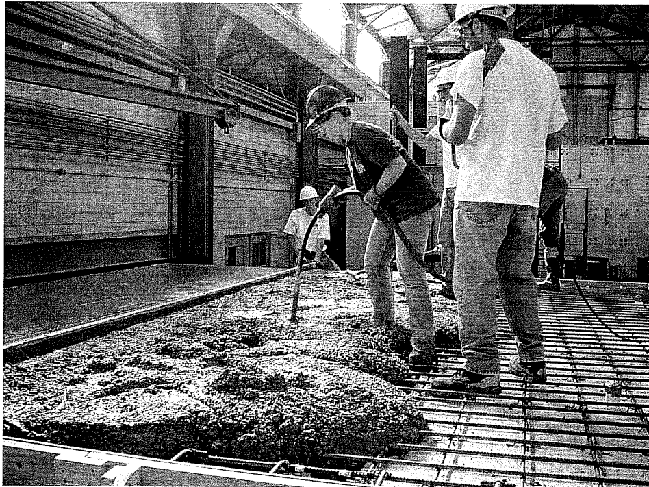
Figure 4.8 Vibrating concrete
