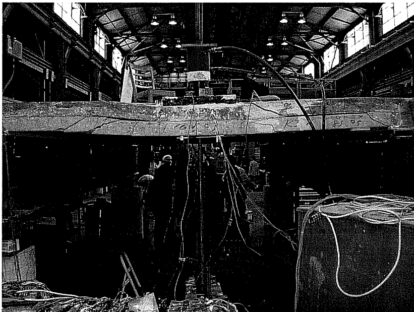
(a) Facing north
